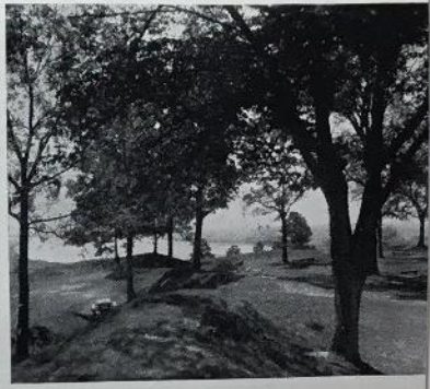
Earthworks of Original Fortifications
