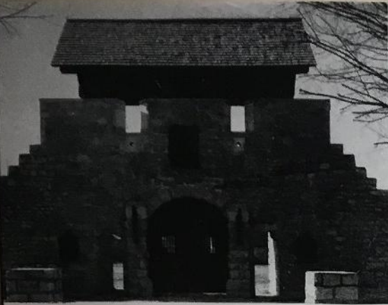
Rebuilt Gateway to Fort Chartres
