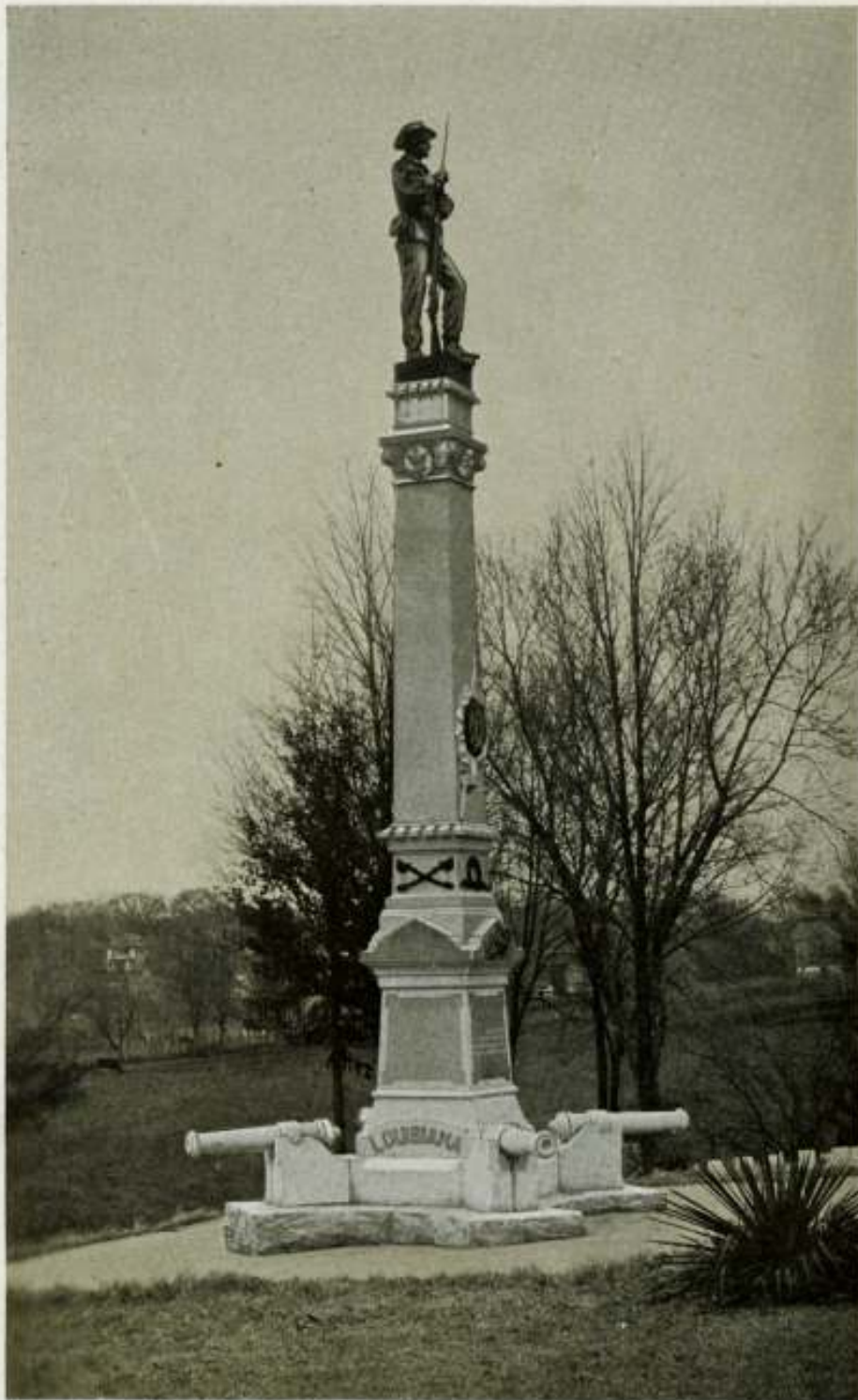
Confederate Soldiers' Monument, Fayetteville, Ark. By F. H. Venn & Co., Memphis, Tenn. Surmounted by 6 ft. statue, No. 5608, page 71. Made in sheet copper, antique bronze finish, by The W. H. Mullins Co., Salem, Ohio.
